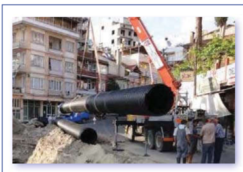
▶ Pipe site installing for municipal projects
