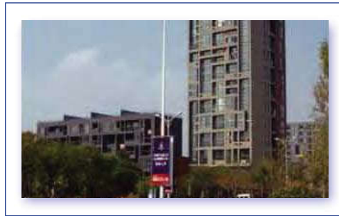
▶ District drainage system in Shenyang
